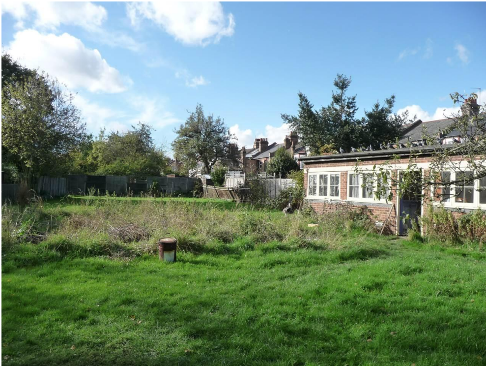
Workshop/shed on the site
